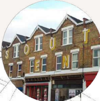
↑ Public welcome: Painted gateway signage on the upper facade of the shops in Croydon Image credit: Spriestersbach
